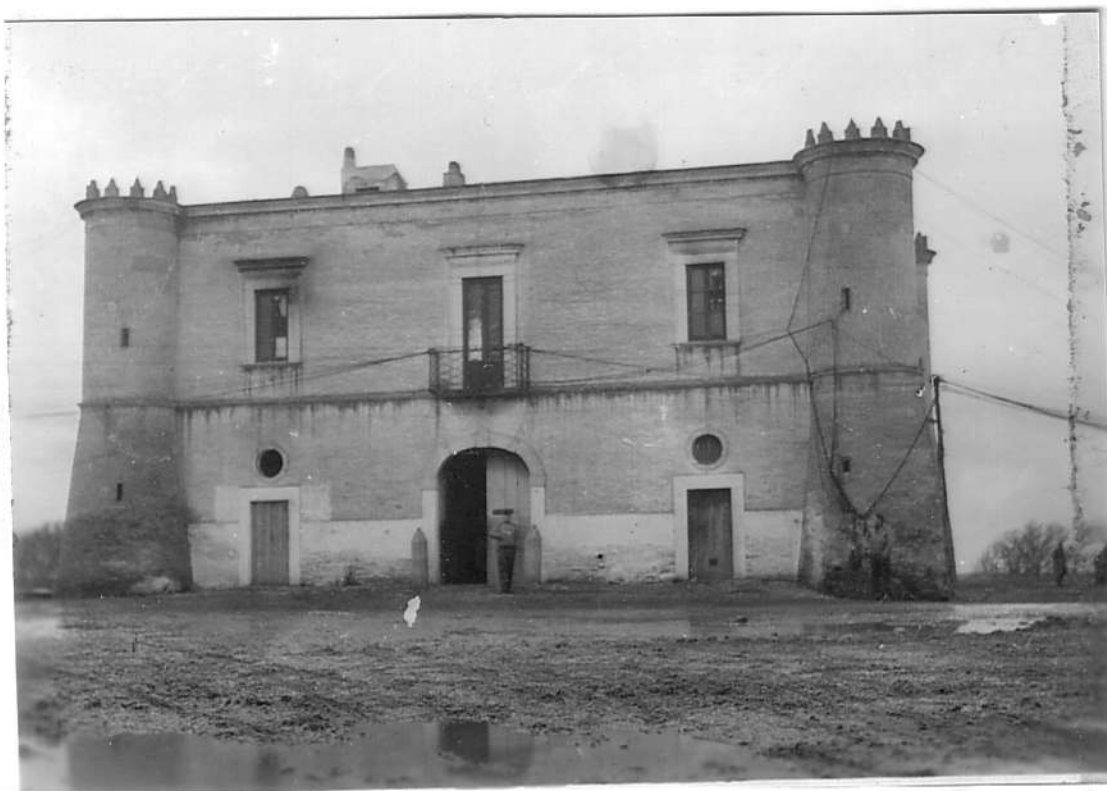
The large door in the middle of the Old Castle is where we had some of our briefing before missions and interrogation after missions. The smaller door on the left was the Red Cross door where they brought out a long table and had a shot of Irish Whiskey, coffee, and donuts after a mission.
