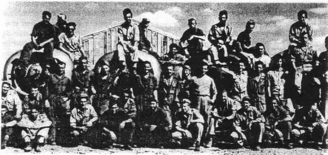
740th Squadron maintenance personnel.
